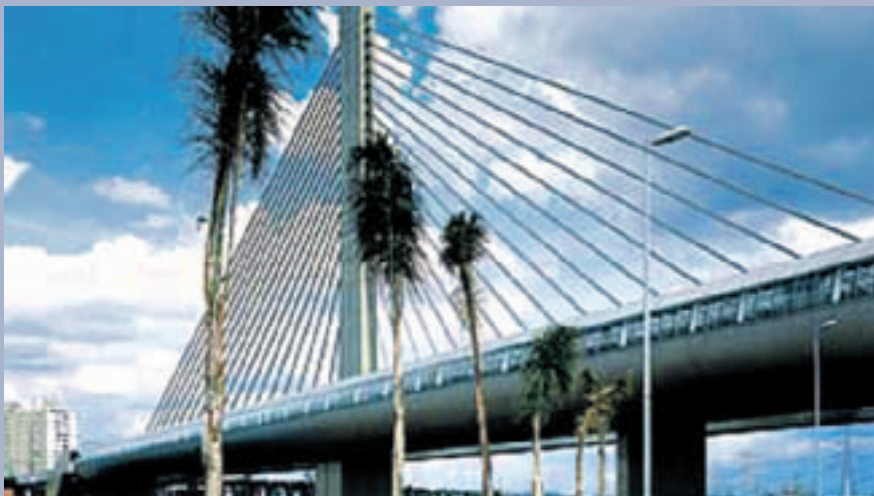
Figure 9: USM® track mats used for a track on a bridge
