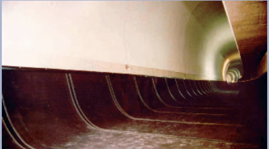
Figure 6: USM® track mats in a tunnel before ballasting
