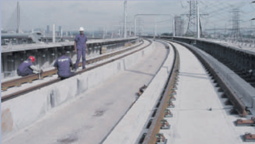
Figure 8: USM® track mats placed under concrete on an elevated track
