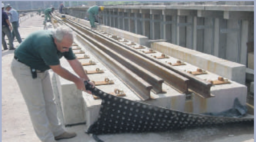
Figure 11: Stripped “light” mass-spring-system with USM® track mats
