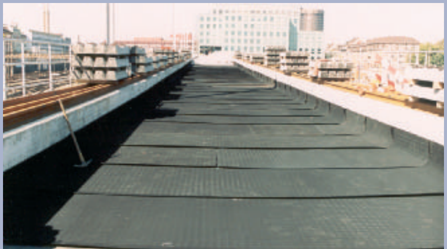
Figure 7: USM® track mats on a concrete bridge before ballasting
