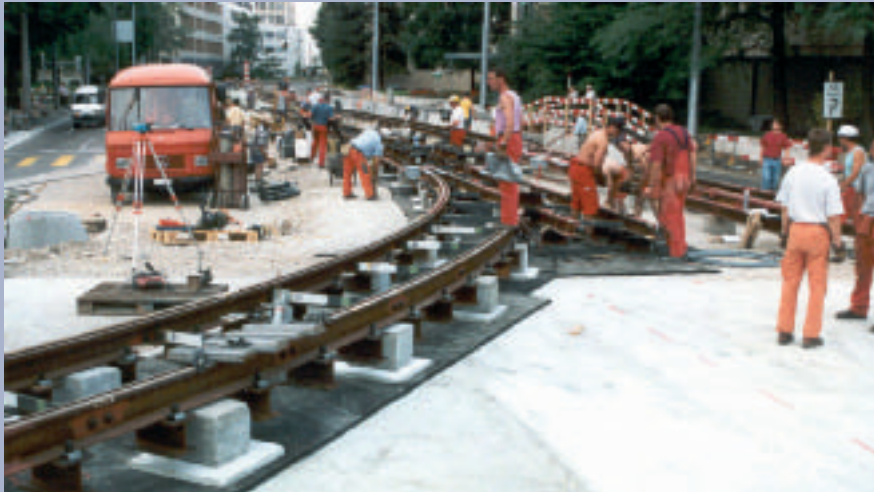
Figure 12: "Light" mass-spring-system with USM® track mats for road tracks
