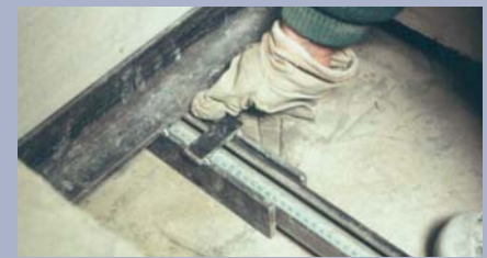
Picture 3: Positioning of the MSS elastomeric Bearings
