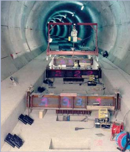
Picture 1: Lifting of the Concrete Element
